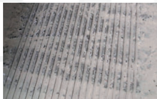
Grooved profiles in concrete surfaces
